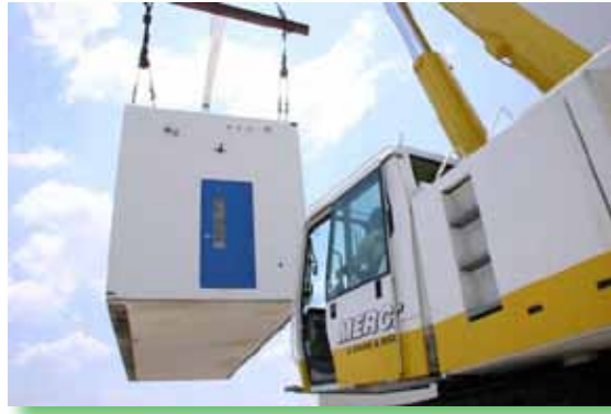
Figure 5 Portable classroom being lifted into place. Photo courtesy of Royal Concrete Concepts, Inc.
