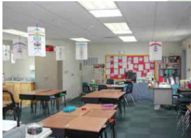
Figure 4. Portable with tubular skylights and electric lights on.
